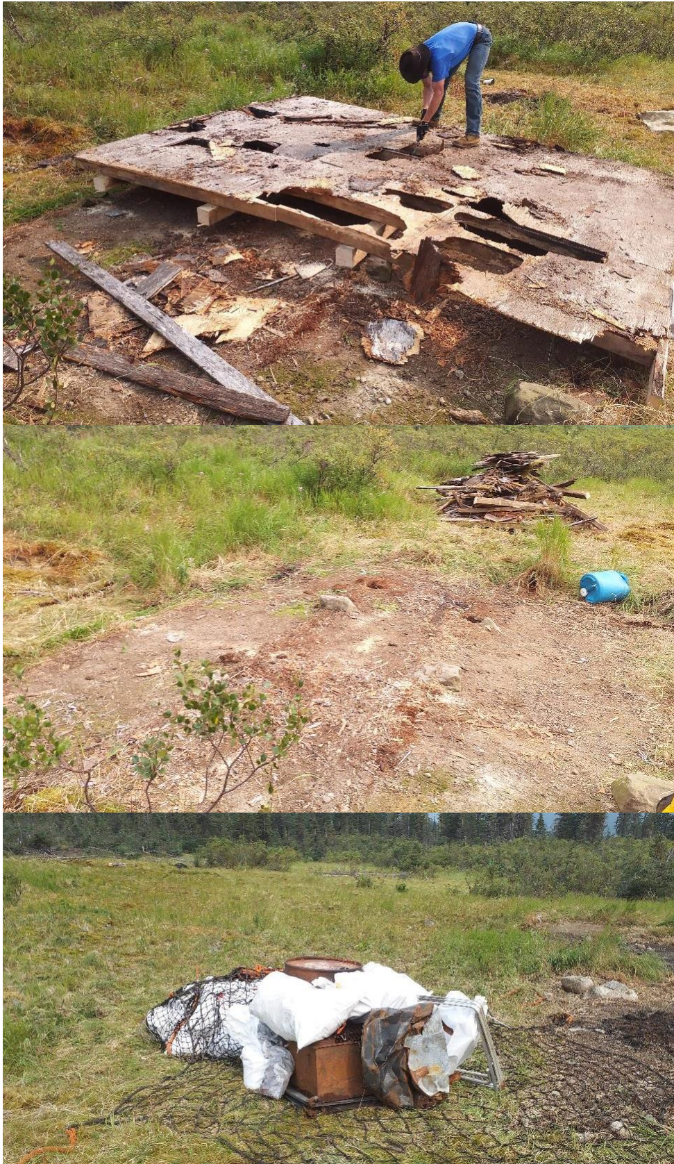
Figure 1 – Reclamation of an abandoned third-party exploration camp on Snowline’s mineral tenure. Top: Site during cleanup – deconstructing a tent platform. Middle: Site following cleanup, before burning of combustible materials. Bottom: Metals and other non-combustible debris were slung by helicopter from site for disposal at proper facilities.
